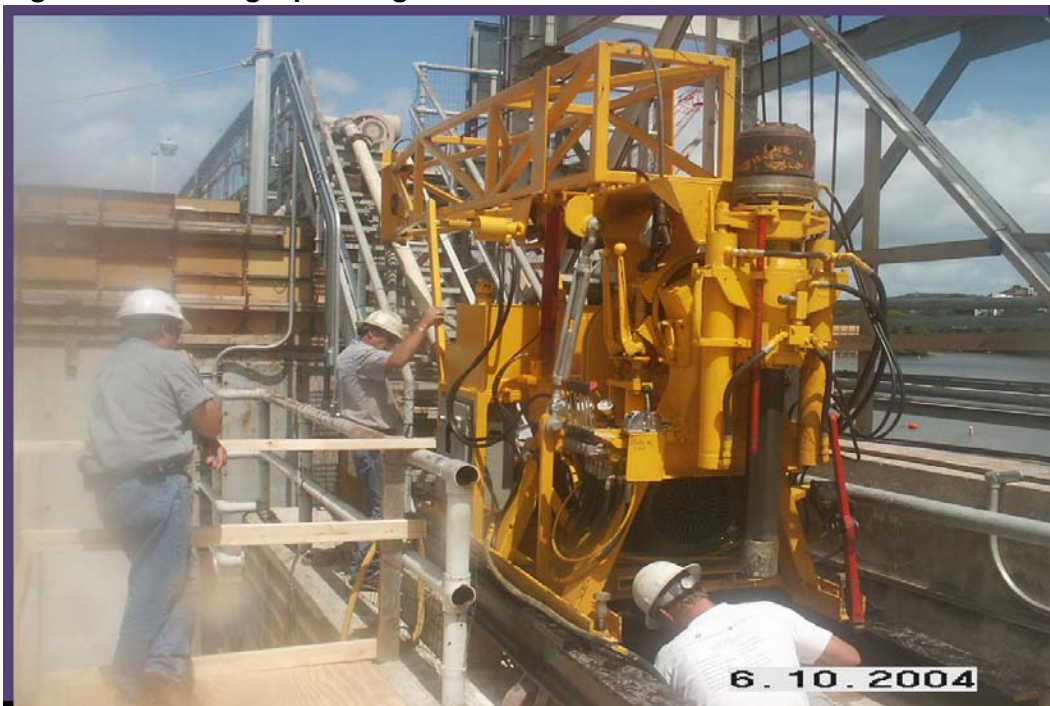
Figure 1 – Drill Rig Operating at Powerhouse Intake
